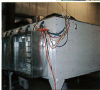
Exterior of the chambers
